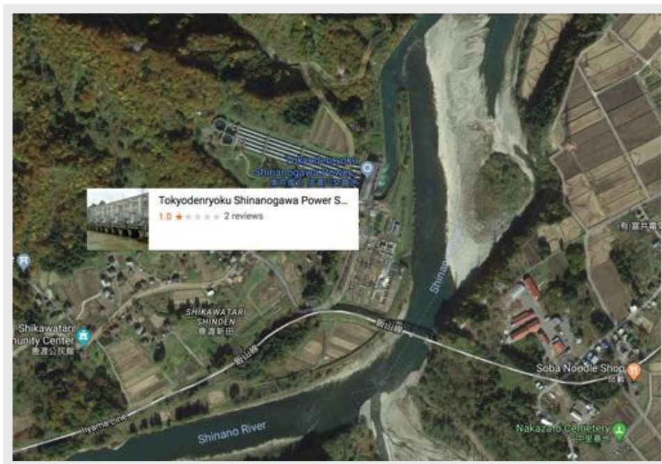
Figure 12. Hydro power plant in Japan
